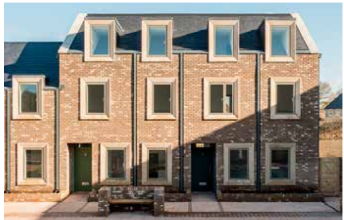
Figure 40 Temple Gardens, Temple Cloud, Bristol. Reinterpretation of traditional forms and fenestration with use of brick and stone window surrounds. A design that feels rooted in place without resorting to pastiche. (Archio)
