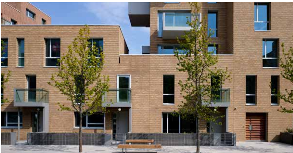
Figure 49 Lower and higher density housing typologies should always address the street directly with door and windows (Allies and Morrison)
