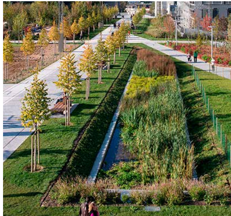
Figure 24 SuDS attenuation basin and swales can create natural boundary edges (Grant Associates)
