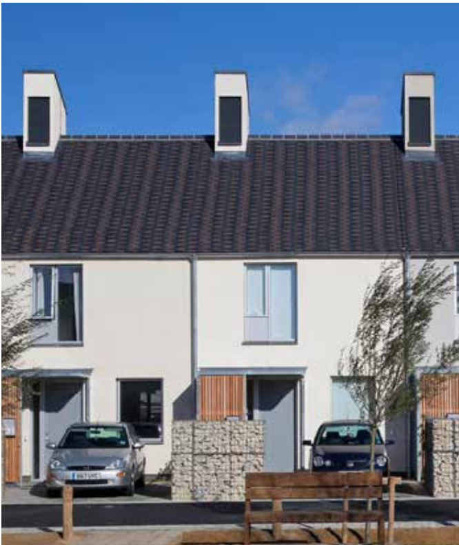
Figure 6 The "Triangle" by Glenn Howells Architects was supported by the Government's Low Carbon Investment Fund. Homes have bicycle storage built in to the front canopy of each house
