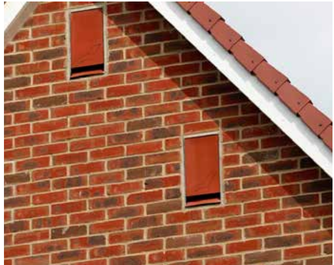
Figure 9 Precedents: Kingsbrook Aylesbury, Set a new benchmark for wildlife friendly housing development. 2,459 homes have been built on greenfield land, and designed so wildlife can move freely through the residential areas. Swift boxes are shown here, built into the roofs of new home
